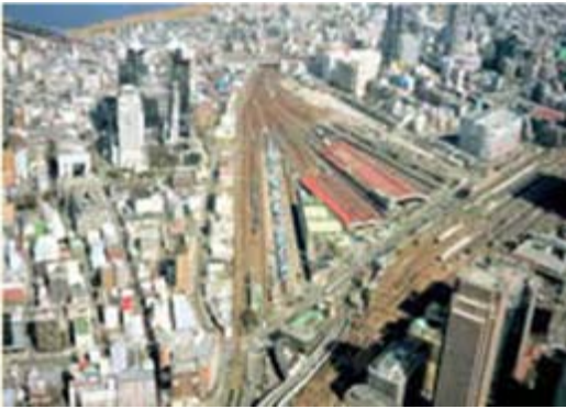
No.1 – Umeda North Yard (The aerial photograph courtesy of Osaka City)
